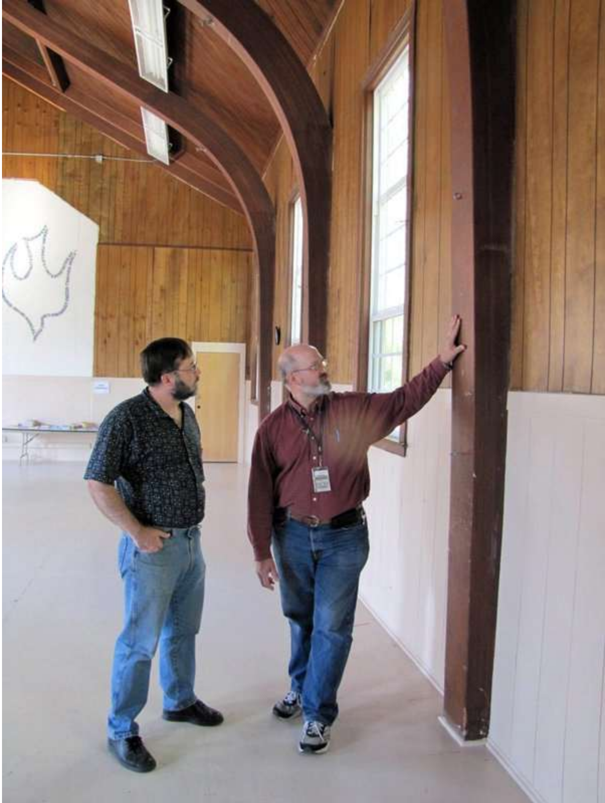
Historian Jeff Davis, left, and Memorial Lutheran Church custodian Jim Wulf examine one of the beams that would have to be braced if the former World War II Army chapel were relocated. A group of military veterans wants to buy the chapel and move it from the church campus to a
